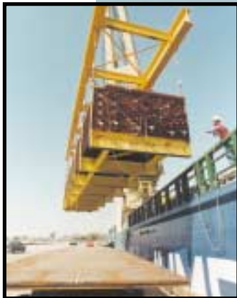
A HRSG module weighing 150 tons is eased over the side of the m.v. Jumbo Vision and placed on board a heavy-duty railcar for shipment to the jobsite in Arkansas.
